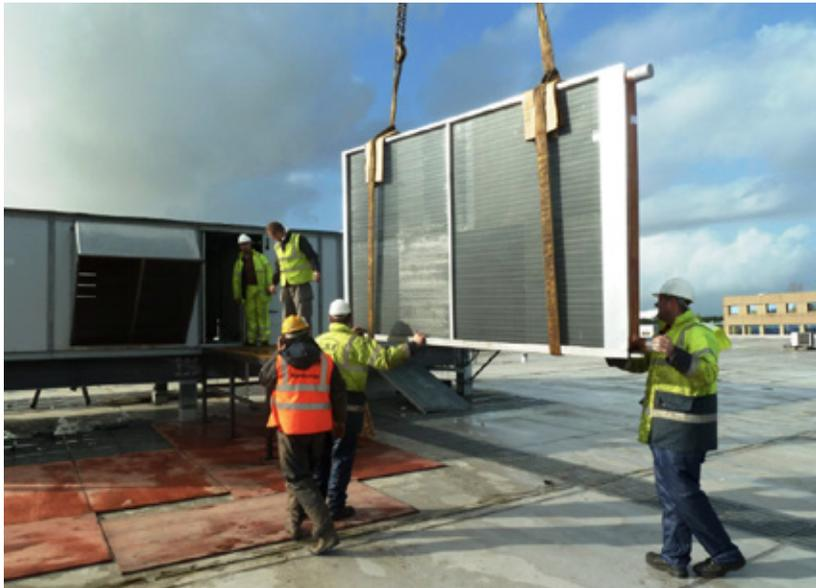
The new heat pump units – mounted on new structural frames with associated buffer vessels, twin pump sets and heat exchanger coils – were individually craned into position and installed over two weekends. The only downtime on the existing roof top units was during the removal of the old DX coil and installation of the new water-based coil.
