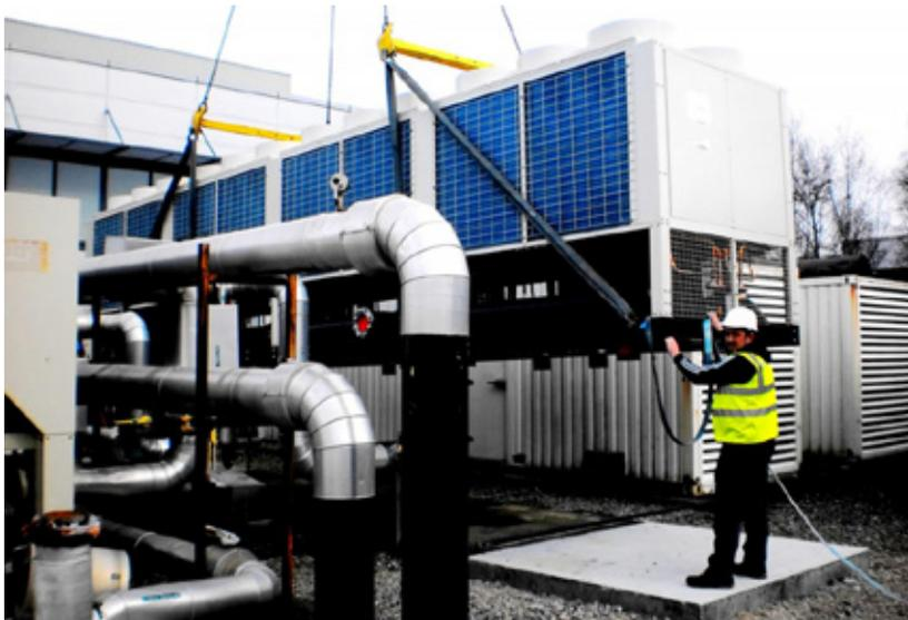
The new chillers models provide modular, individual refrigeration and hydraulic circuits utilizing low noise and vibration modulating compressor technology and high efficiency plate heat exchangers, optimized for use with ozone friendly refrigerants R407c.
